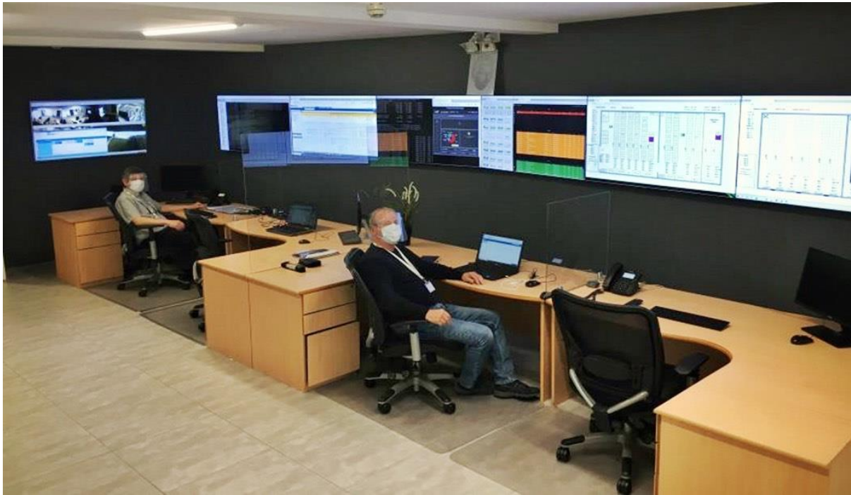
Figure 1 24/7 x 365 Network Operations Centre
